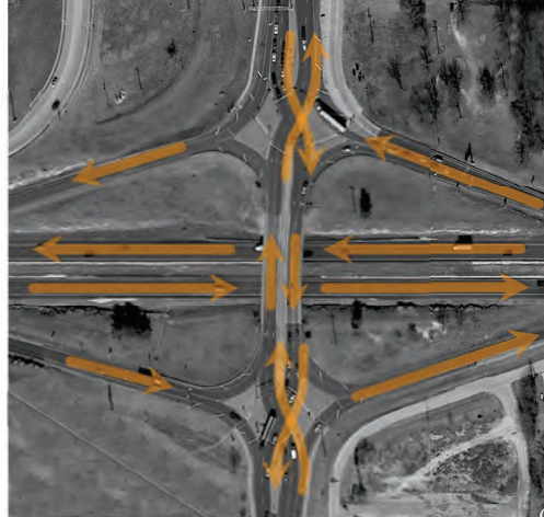
DIVERGING DIAMOND INTERCHANGE WITH ACCESS TO AND FROM BOTH SIDES OF SR 836
