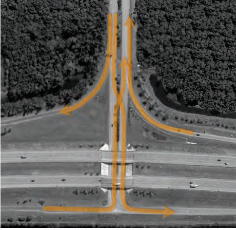
PARTIAL DIVERGING DIAMOND INTERCHANGE WITH ACCESS TO AND FROM ONE SIDE OF SR 836
